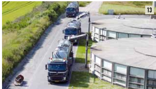
Figure 13: Storage tanks for digestate, covered with concrete tops, at Lemvig AD plant in Denmark. Source: Lemvig Biogas ( www.lemvigbiogas.com )
