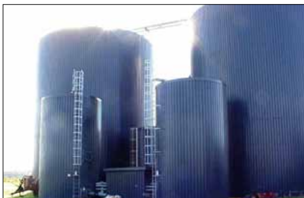
Figure 8: Pasteurisation tanks in foreground, at Blaabjerg AD plant in Denmark. Source Blaabjerg Biogas ( www.blaabjergbiogas.dk )
